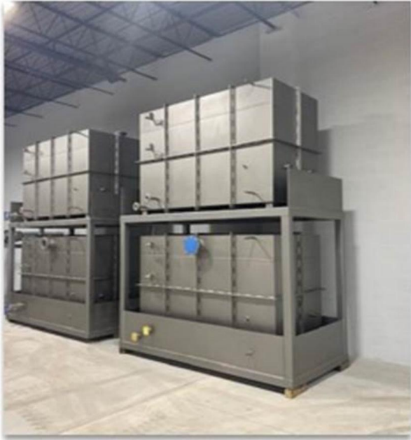
Figure 15. Bubbling scrubber.
